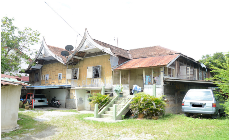
Figure 2. Renovated and extended (including building rooms with brick walls under the original on stilts traditional house) Traditional Malay House of Kelantan at Kota Bharu, Kelantan, Malaysia.
